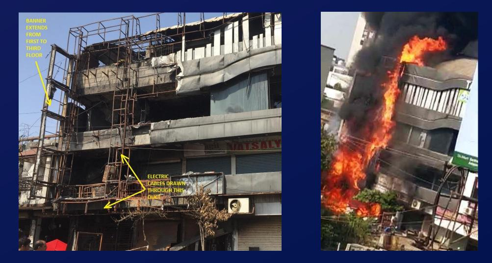
Heat from initial fires ignited banner and the cable duct, and travelled to the fourth floor (other floors relatively unaffected)
