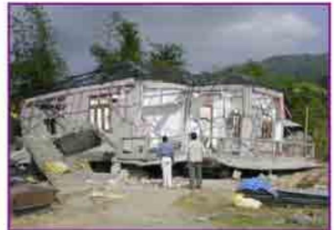
Antitopof two-story 2C frame building with open first floor during 2004 Sumatra earthquake
