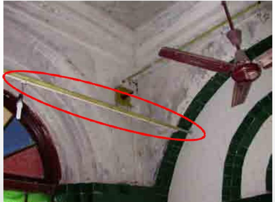
**Tie-rods placed in both directions**
