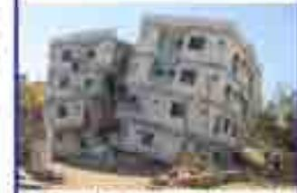
(b) Collapse of moment-resisting columns and building during 2011 Mw 9.0 earthquake
