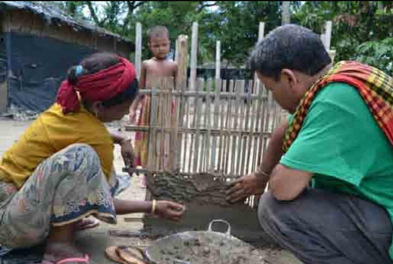
Wattle and daub wall with bamboo and cement stabilized soil
